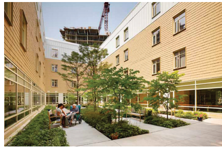
The Wellesley Central Place, a division of the Drs. Paul and John Reka Centre, is unlike any other long-term care home in Toronto. Designed to function as an independent village, it emphasizes wellness focusing on the capabilities of individual patients, rather than a disabilities-centred medical model.
